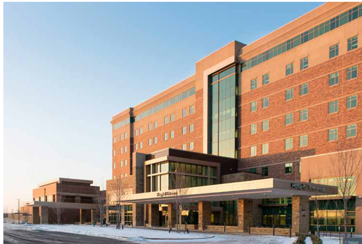
Contractors such as McCarthy Building Cos. use techniques such as prefabrication to accelerate the construction process. Pictured is Mercy Hospital Joplin, an 890,000-square-foot hospital in Joplin, Missouri, that McCarthy constructed in 46 months.
